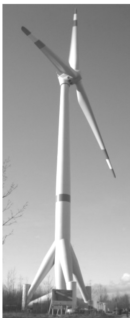
Figure 10: 5 MW Multibrid 5000 off-shore wind energy plant as on-shore prototype.
